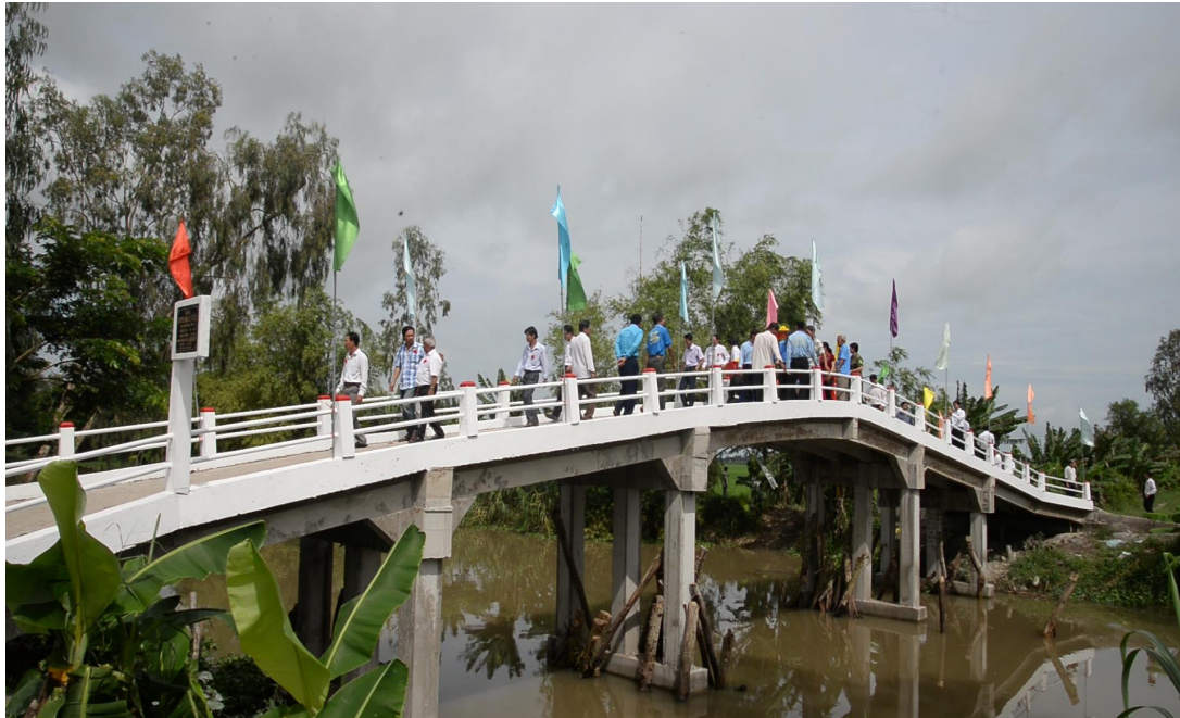
Figure 7.5 A concrete bridge constructed by Hoà Hảo builders.
