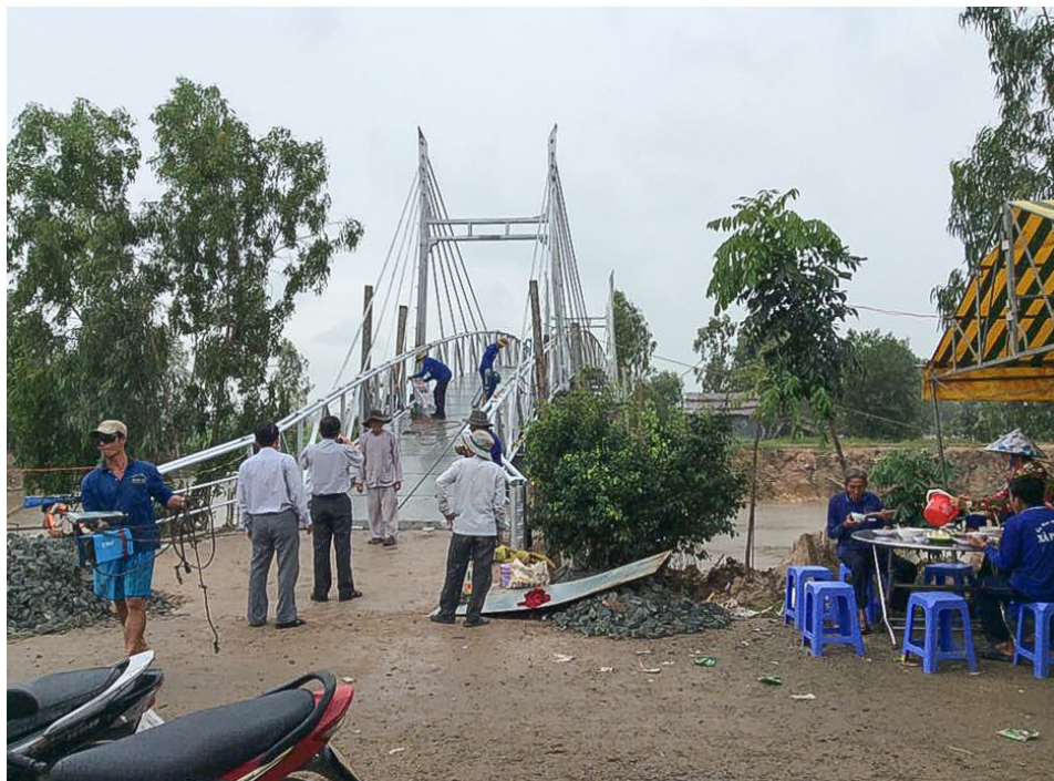
Figure 7.1 A steel, cable-stayed bridge built by Hoà Hảo Buddhists.
