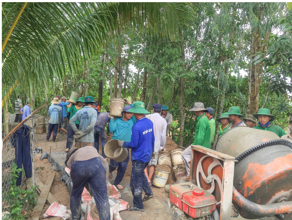
Figure 7.2 Hoà Hảo Buddhists working at the construction site.
